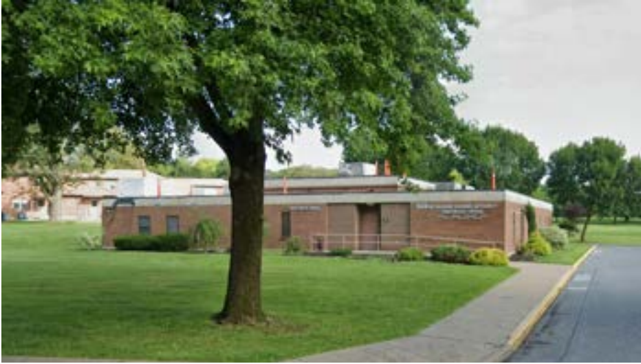
1. Bethlehem Housing Authority: Northeast Office
