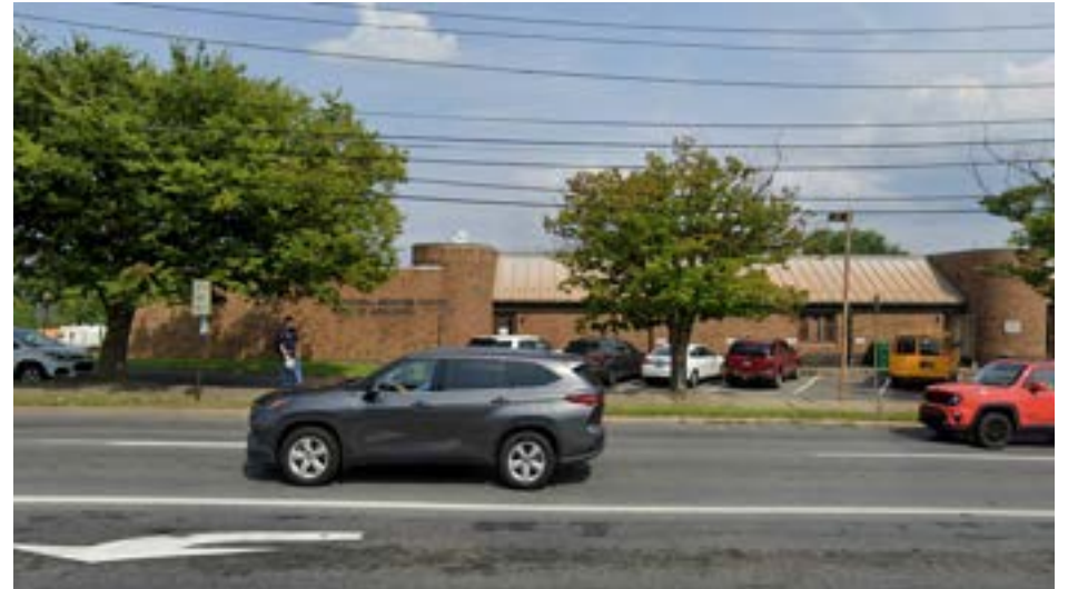
4. City of Bethlehem Municipal Services Center
