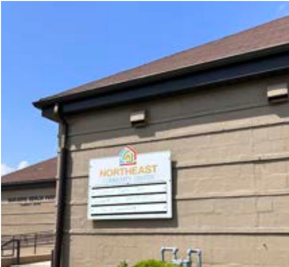
8. Northeast Community Center
