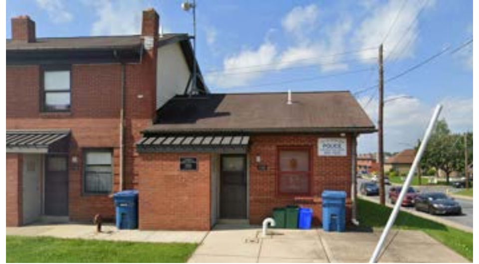
2. Bethlehem Police Department Northeast Sub Station
